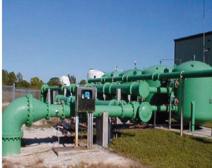
*The pretreatment component of a brackish groundwater reverse osmosis treatment facility. Such a facility could someday be developed in the planning region to desalinate water from the Lower Floridan aquifer.*
